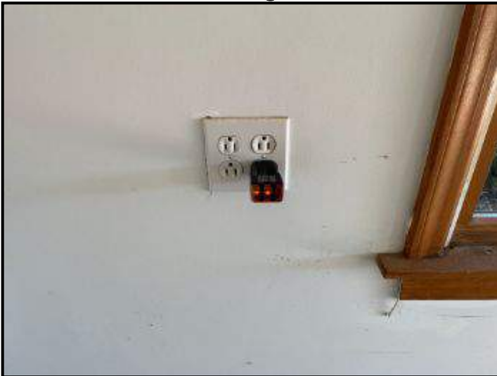
Grounded non-GFCI outlets at garage
