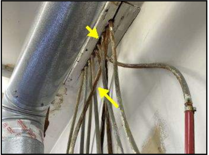
Brown staining at ceiling/down pex water tubing
