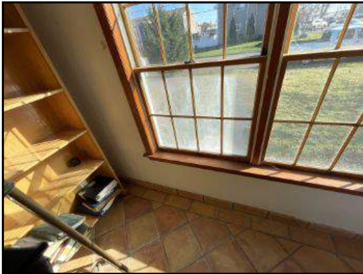
Moisture between panes at lower front living room window
