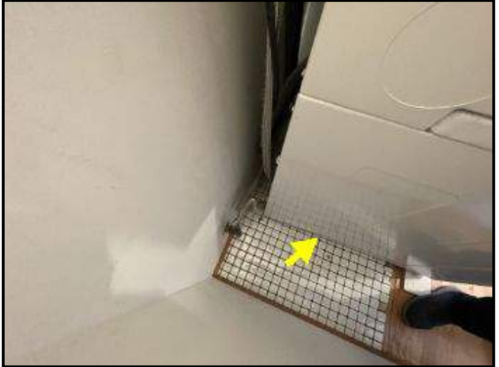
No pan beneath washer/dryer for potential leak
