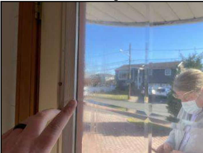
Moisture between panes at front storm door
