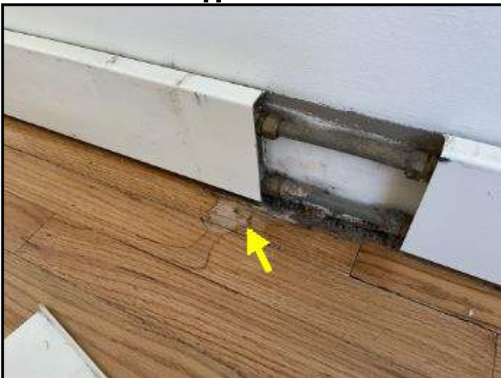
Evidence of past leak at rear upper bedroom baseboard pipe connection; no current leak observed
