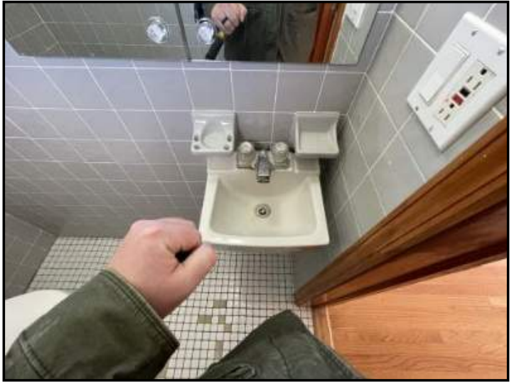
No running water at upper ensuite bathroom sink/toilet
