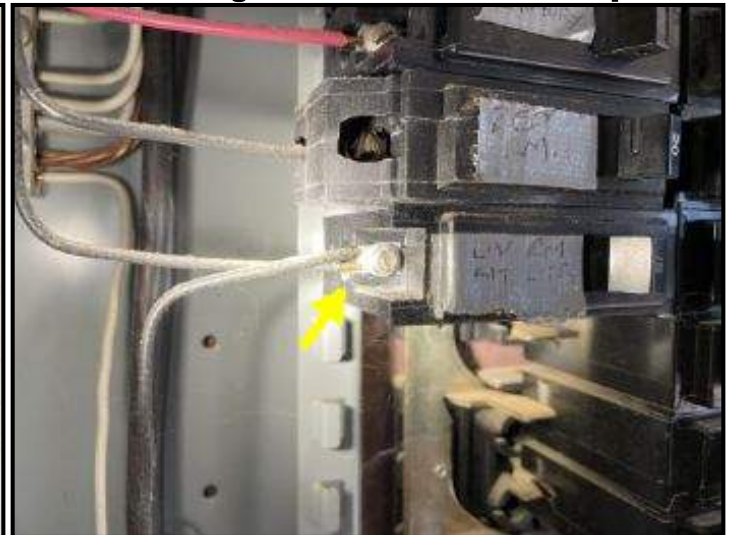
Double-tapped breaker at upper level service panel
