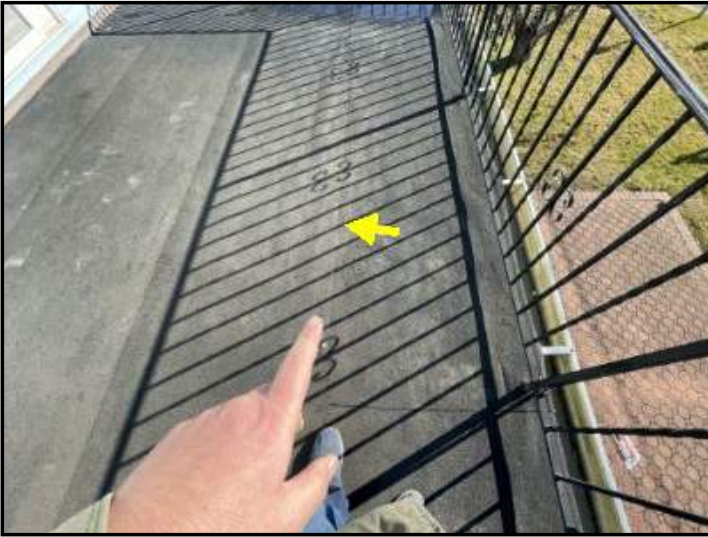
Some areas of flat roof roofing at upper balcony bubbled/soft
