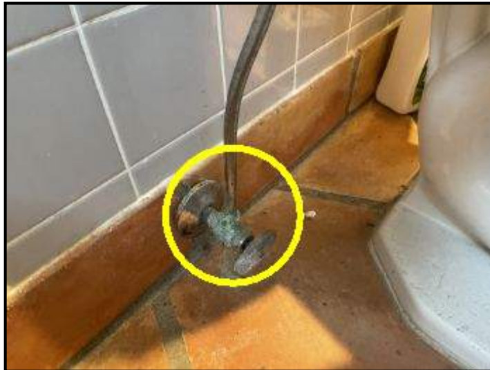
Some corrosion observed at lower main bathroom toilet supply valve
