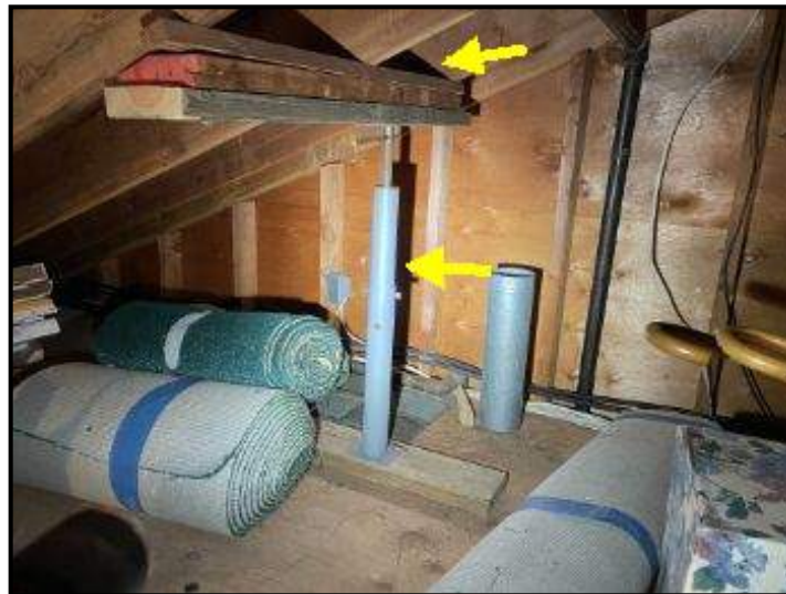
Adjustable column stabilizing roof rafters above garage
