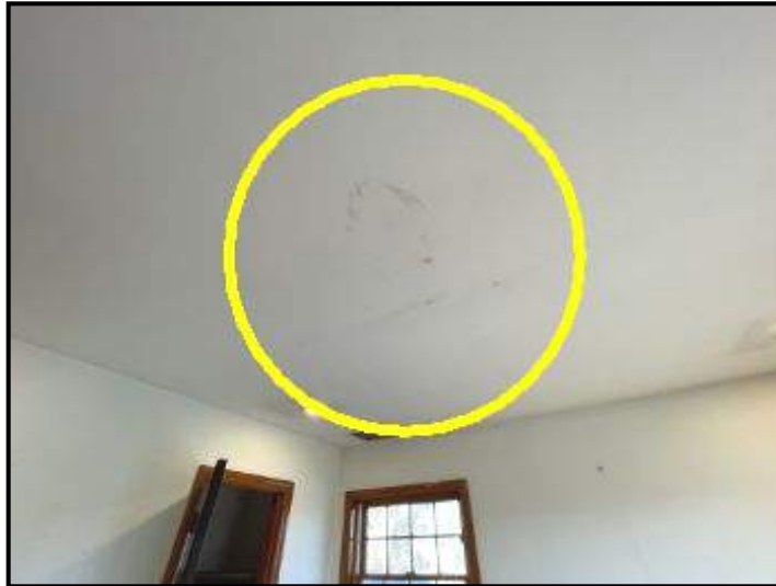
Cosmetic marks/bubbled paint at center of upper front bedroom ceiling; no current moisture observed
