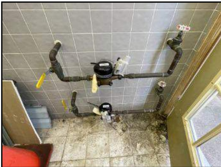
Upper and lower level water main and shut-off
