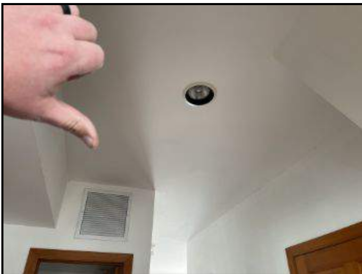
Hallway ceiling light did not operate
