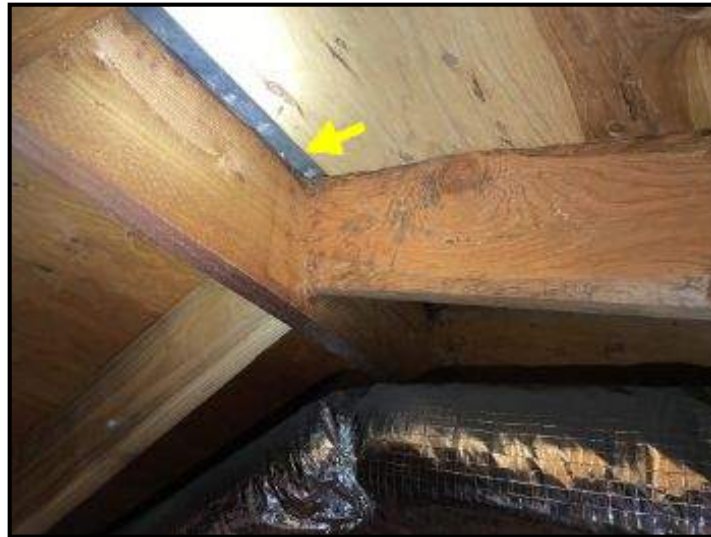
Ridge vent at main roof ridge
