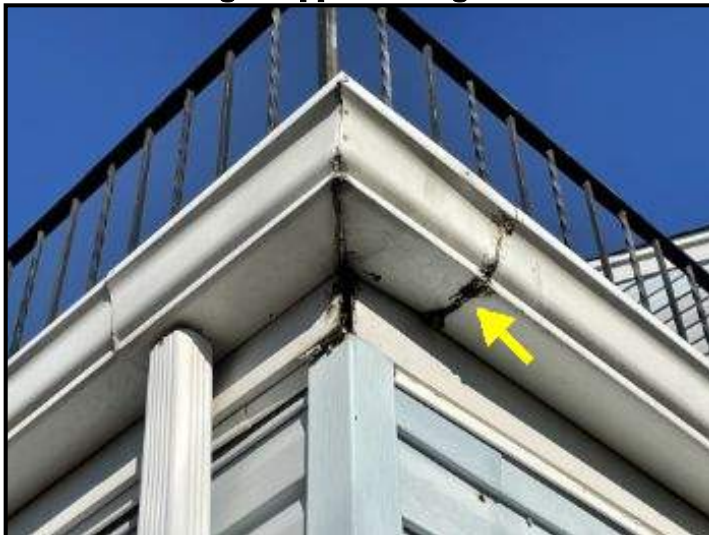
Balcony gutter leaking at gutter seam
