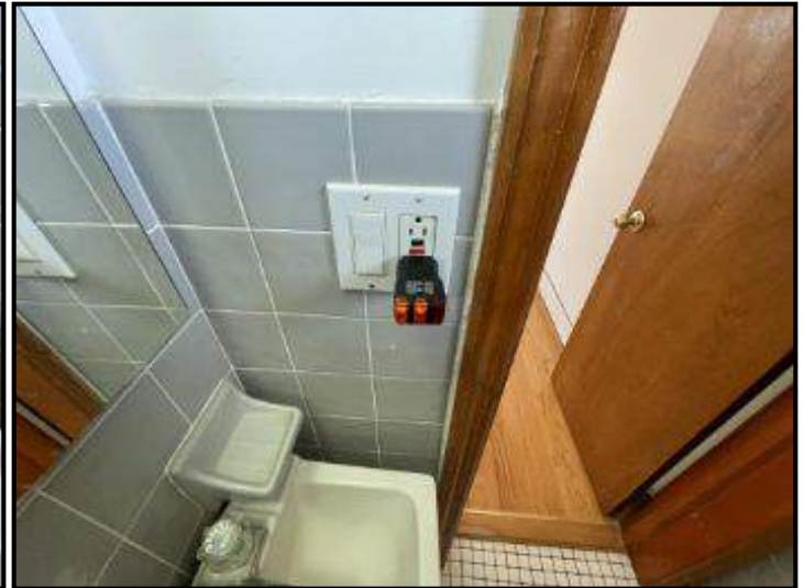
Grounded GFCI outlet at upper ensuite bathroom
