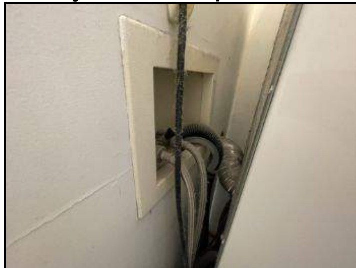
Washer supply/discharge lines
