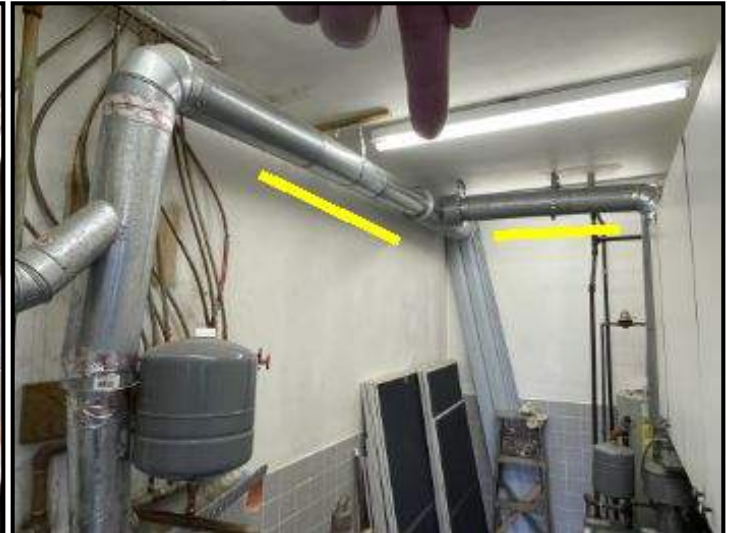
Boiler exhaust vents appeared flat and significant length
