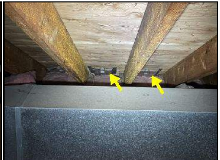
Baffles present at edge of roof for adequate ventilation in attic
