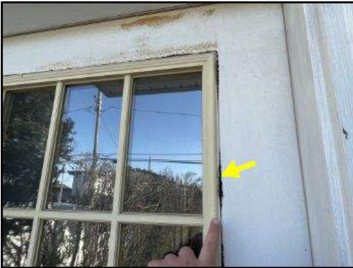
Incomplete caulking around rear door window framing
