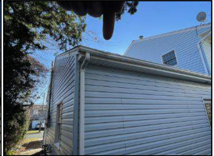
Rear lower gutter sagging
