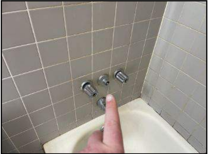
Missing faucet handle at upper main bathroom tub
