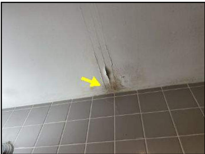
Apparent previous moisture stain at upper main bathroom ceiling; no current moisture observed
