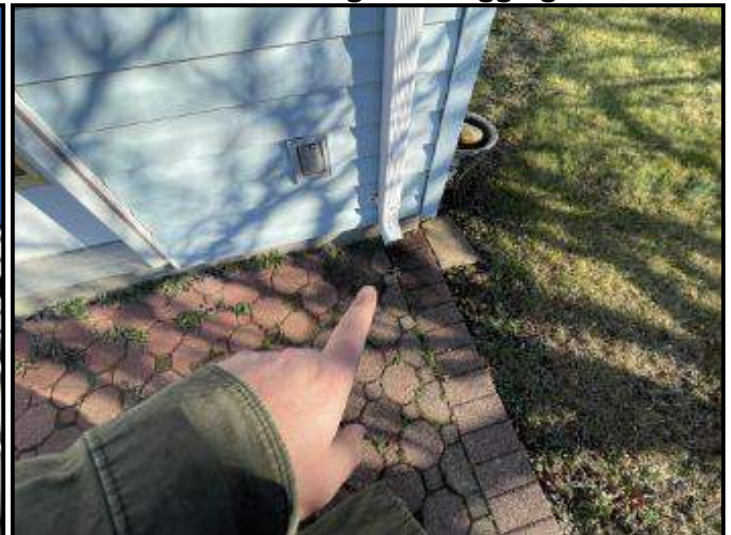
No extensions at gutter downspouts around the home
