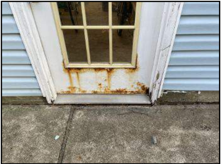
Significant rust at rear garage door
