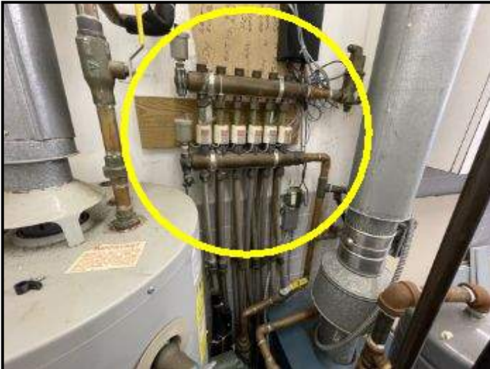
Radiant heat manifold for lower level
