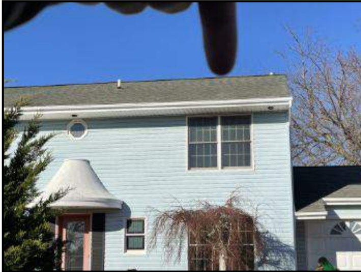
Sag in upper front gutter
