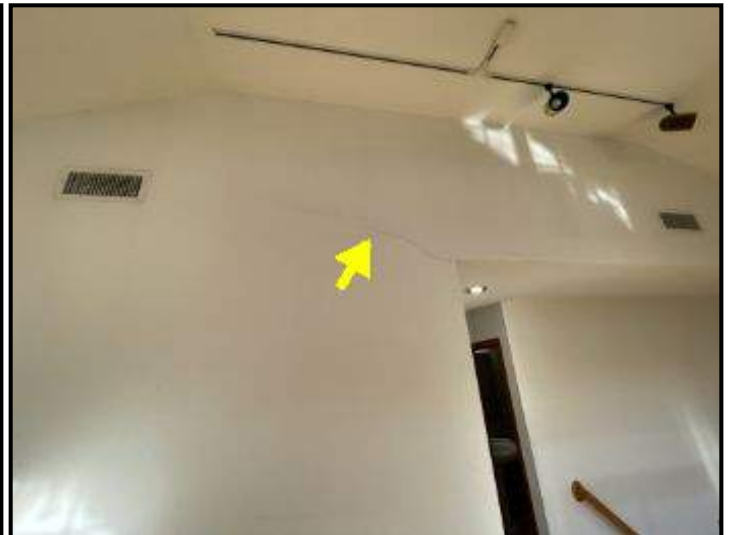
Cosmetic crack/seam at upper living room wall
