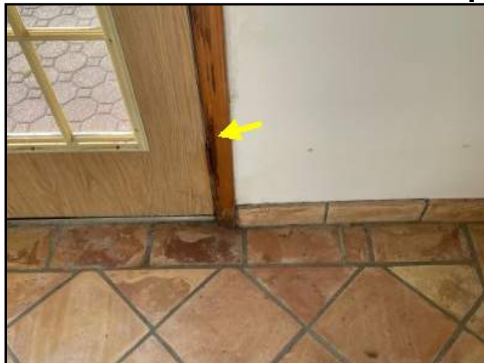
Moisture stains observed around side double door trim at main living room/office
