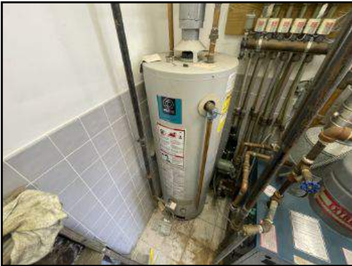
Lower level hot water heater; did not operate
