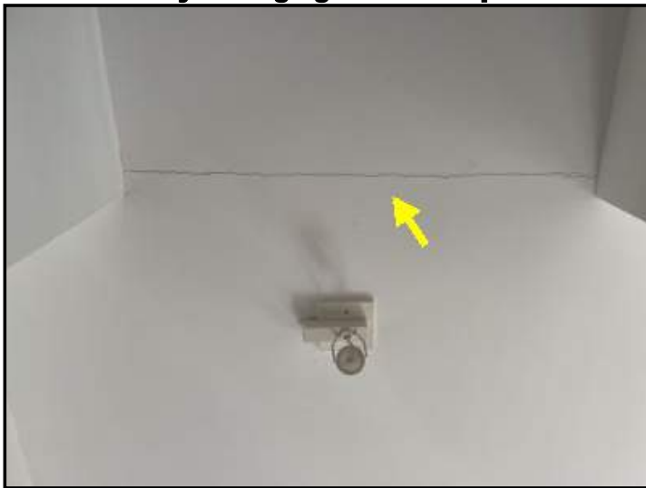
Cosmetic seam at lower hallway ceiling
