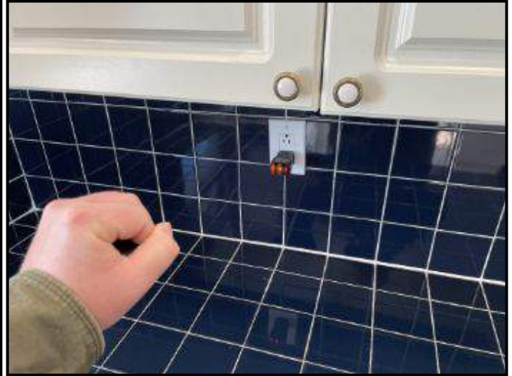
Grounded non-GFCI outlet at kitchen in series with GFCI outlet
