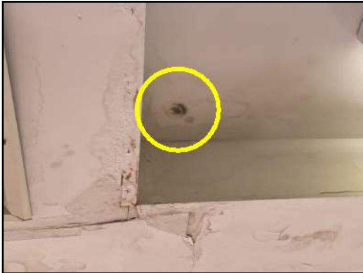
Possible mold at lower main living/office room ceiling near air duct
