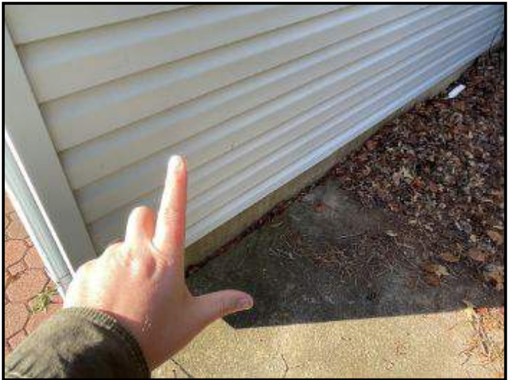
Area of siding not properly secured at side of home
