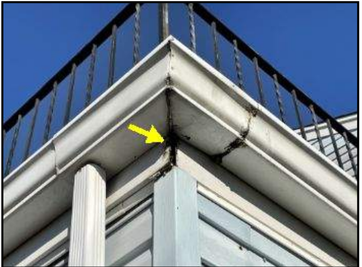
Void at corner of fascia trim at edge of balcony
