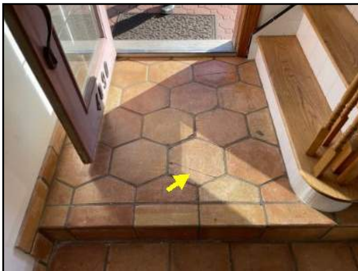
Cracked tiles at front entrance
