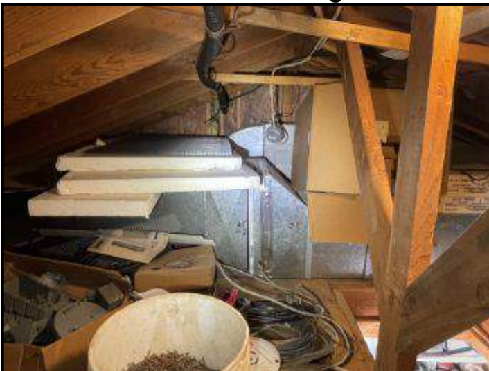
AC evaporator in garage attic
