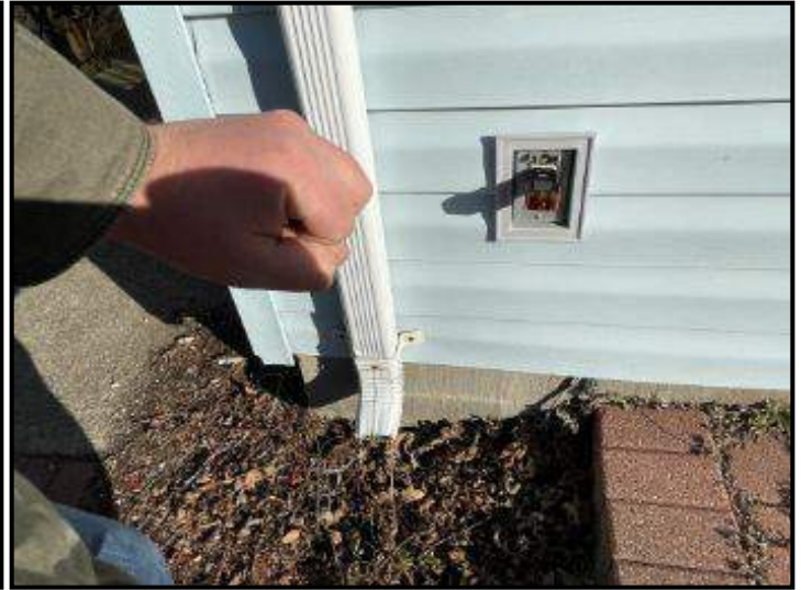
Non-energized outlet at side of home
