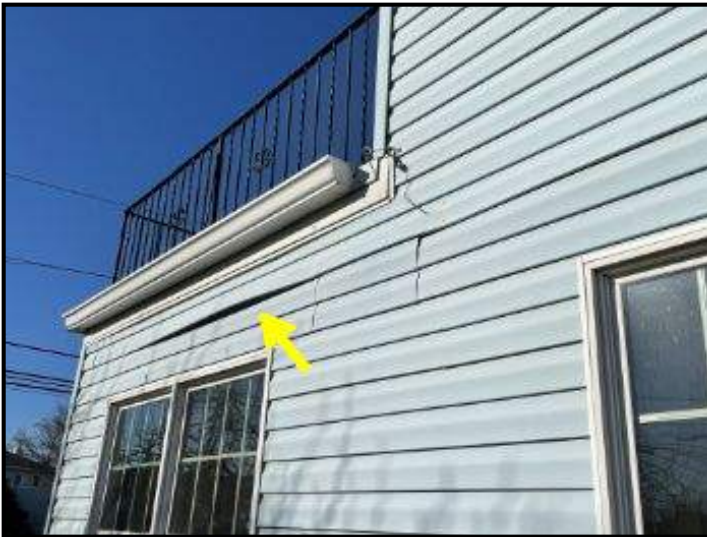
Siding not properly fastened at front of home; appears previously patched
