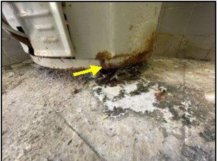
Rust around base of hot water heater
