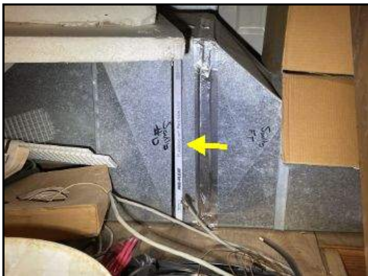
Air filter at Evaporator
