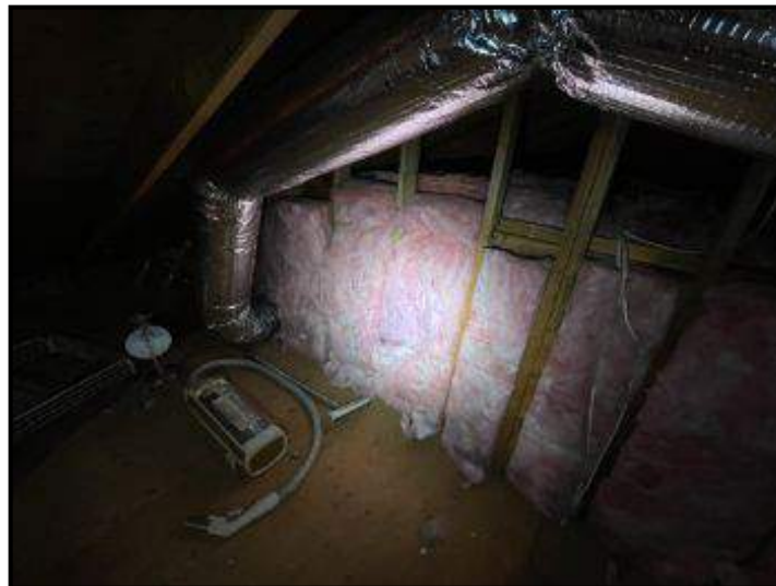
Insulation at vaulted walls/ceiling in attic
