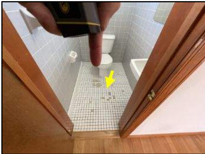
Low area in floor at upper ensuite bathroom
