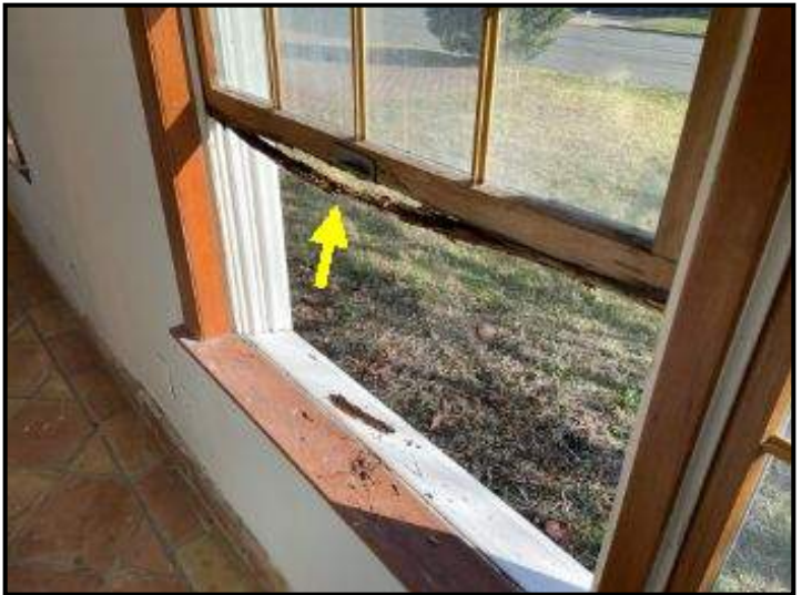
Deteriorated base of lower main living room/office window frame
