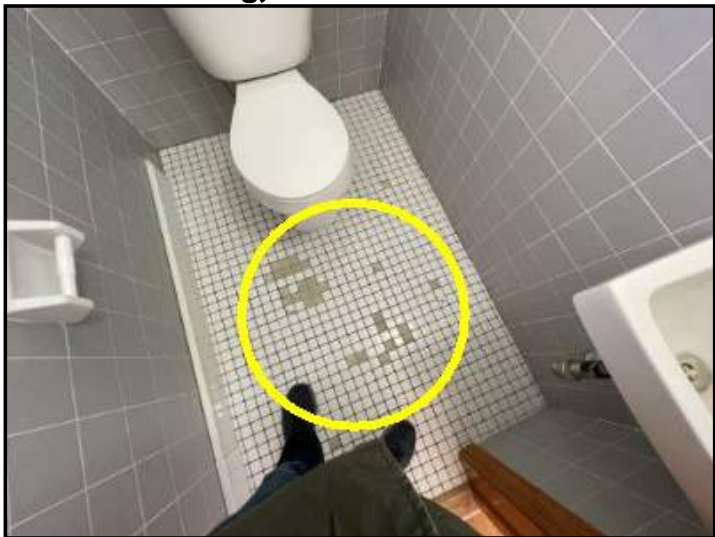
Some missing floor tiles at upper ensuite bathroom
