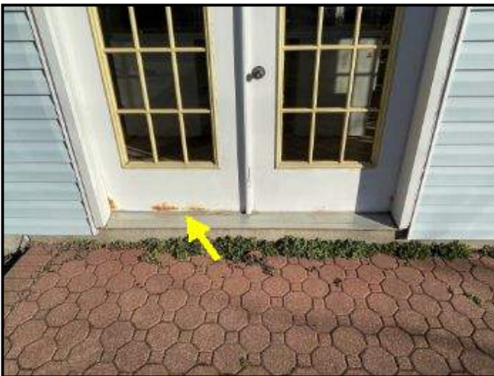
Rust observed at lower portions of exterior doors
