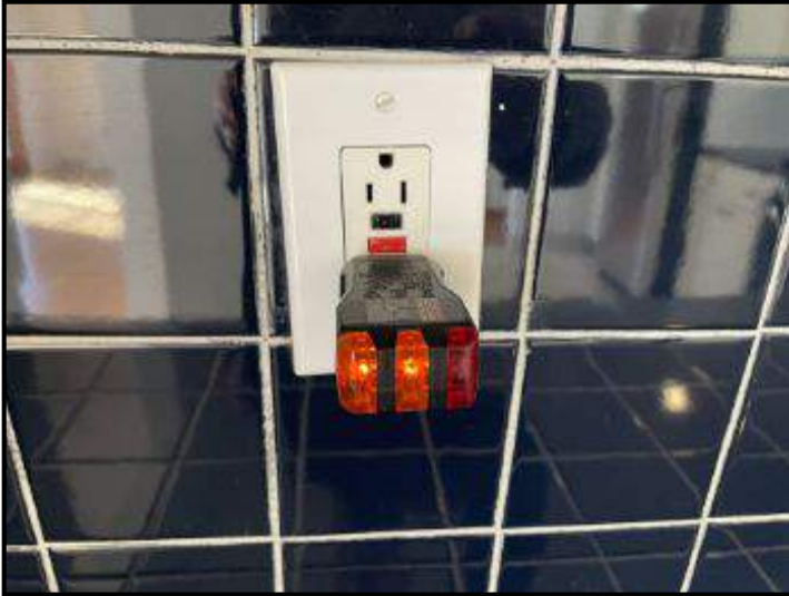
Grounded GFCI outlets at kitchen
