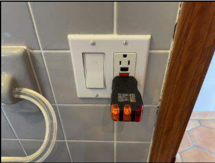
Grounded GFCI outlet at lower main bathroom
