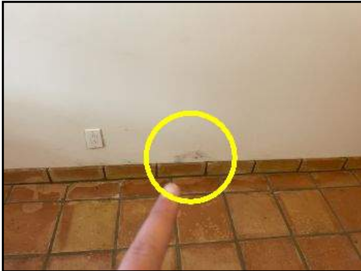
Possible mold at lower rear office wall
