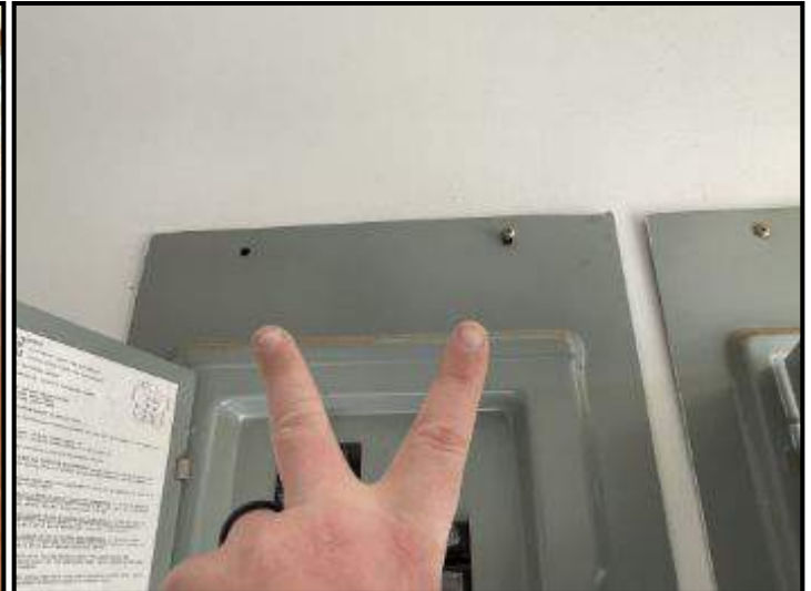
Some missing/loose screws at service panel
