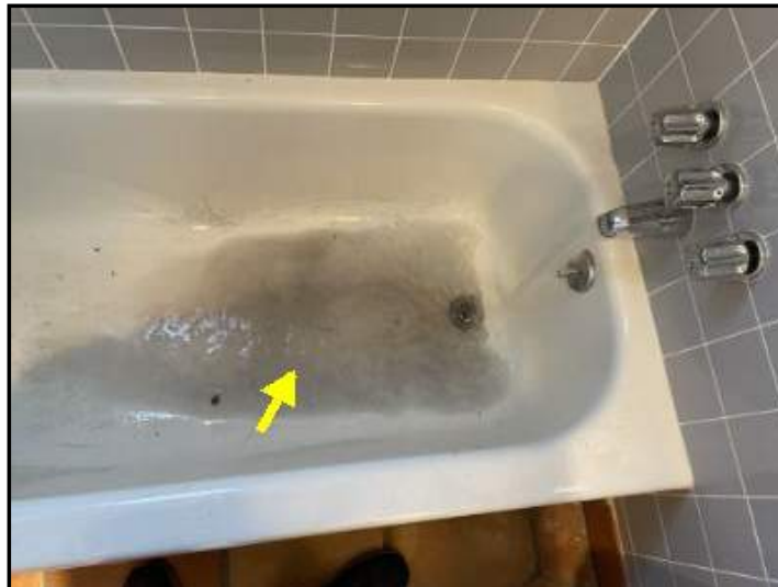
Discolored water at lower main bathroom tub
