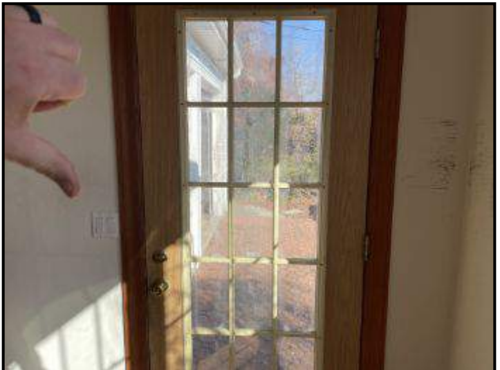
Moisture between panes at front-side door
