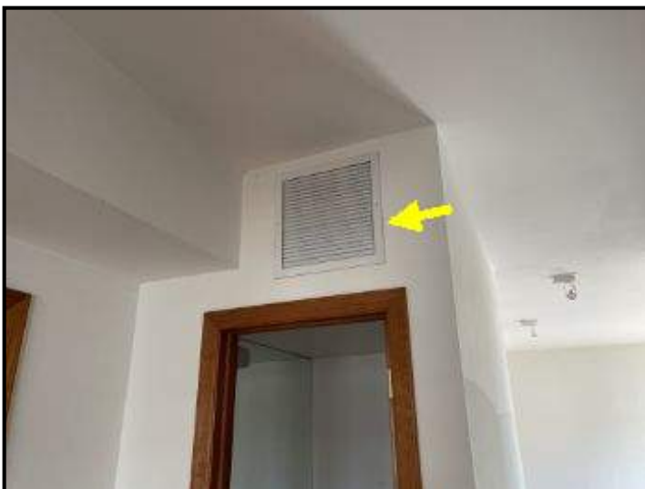
Return air grill at lower hallway
