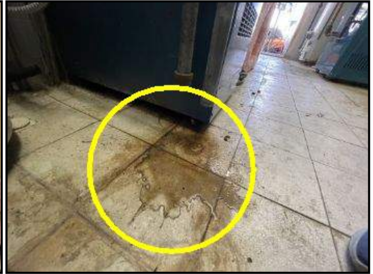
Moisture observed beneath lower level boiler pressure relief valve
