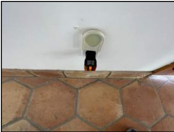
Non-grounded outlet at lower hallway
