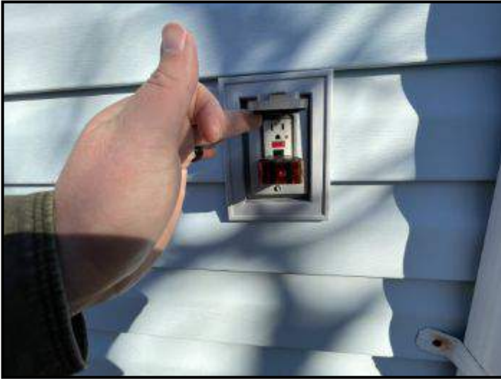
Grounded GFCI outlet at side of home
