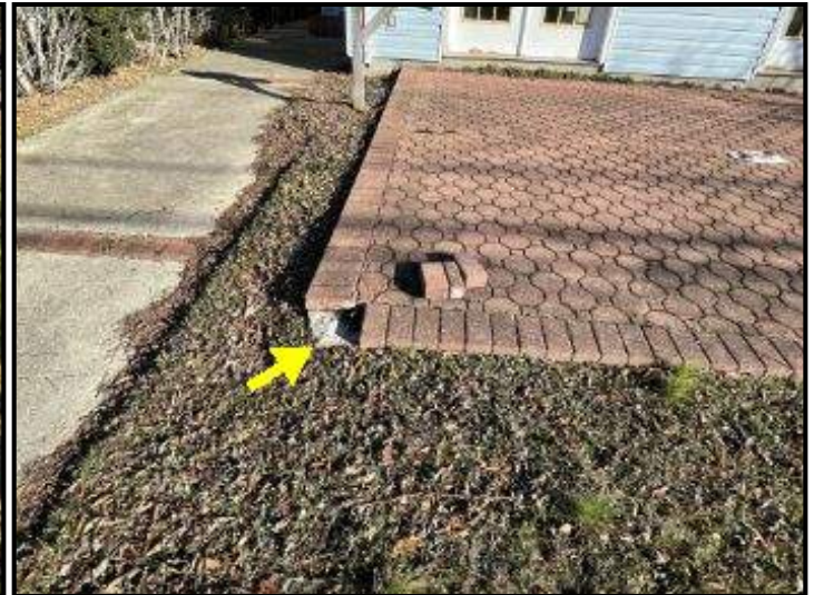
Some pavers at perimeter of side patio were not properly secured
