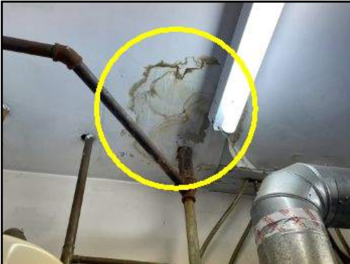
Brown staining around water piping above boiler; no current moisture observed
