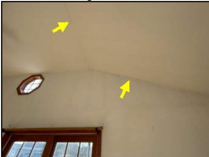
Cosmetic seams at upper living room wall/ceiling joints
