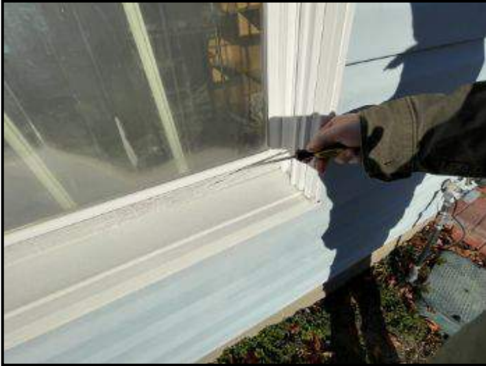
Rotted/deteriorated trim at base of front lower windows
