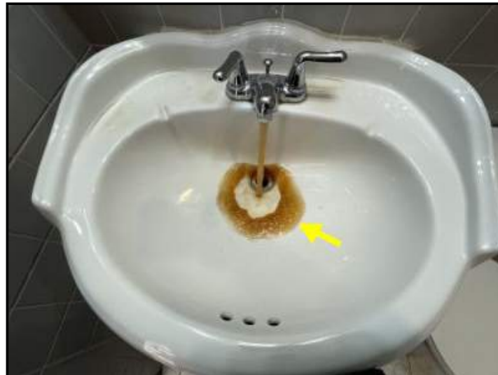
Discolored water at upper main bathroom sink
