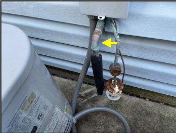
Areas of suction line missing insulation
