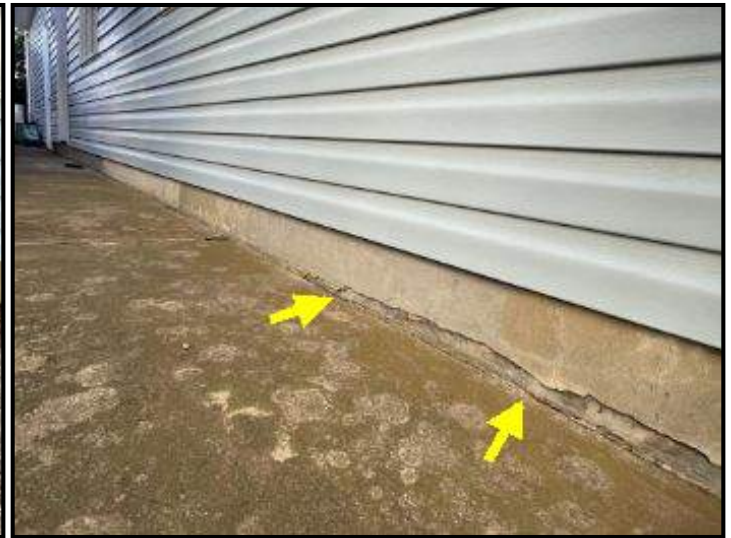
Cracked concrete parging at several areas around the home
