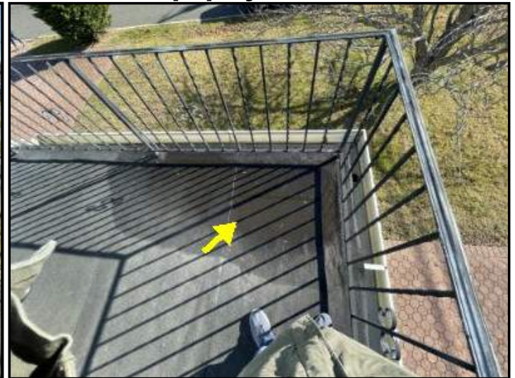
Low area at edge of upper balcony; standing water observed
