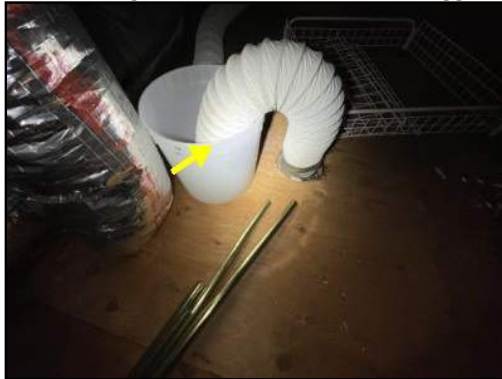
Main upper bathroom exhaust fan does not discharge to exterior
