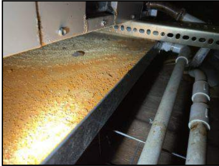
Rust observed at AC evaporator pan; no float shut-off switch encountered
