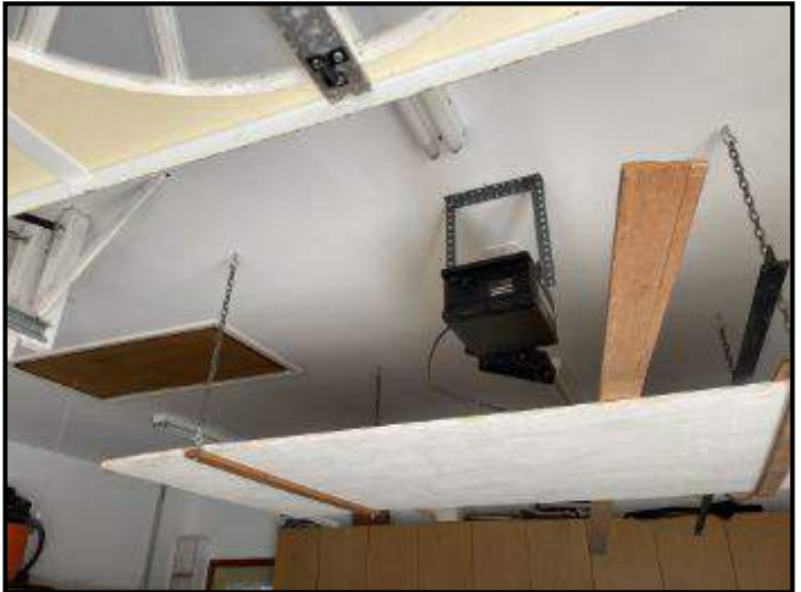
Automatic garage door opener disconnected
