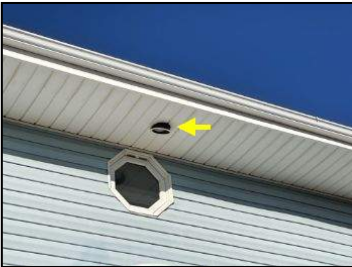
Exterior lights at front eave not properly secured
