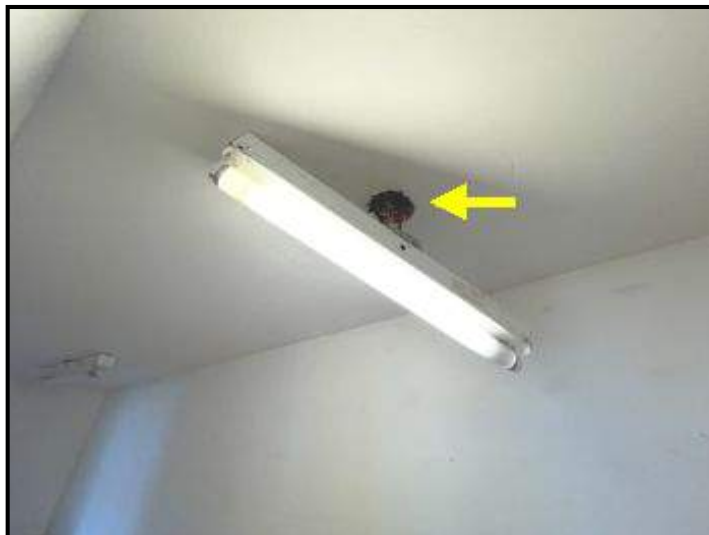
Upper front bedroom closet light not properly fastened to ceiling
