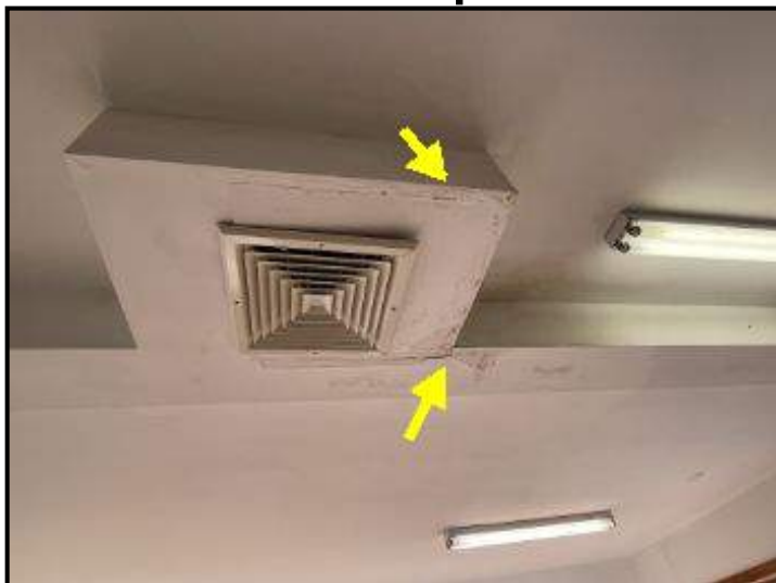
Moisture stains observed at air ducts above lower main living/office room
