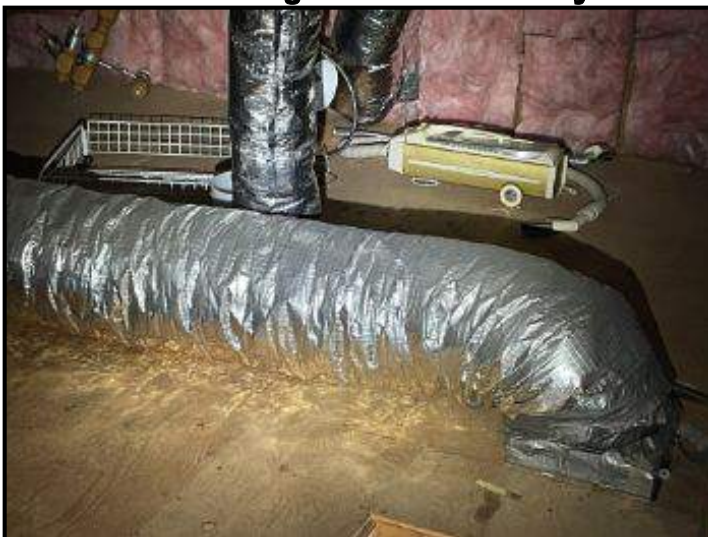
Insulated AC ducts throughout attic
