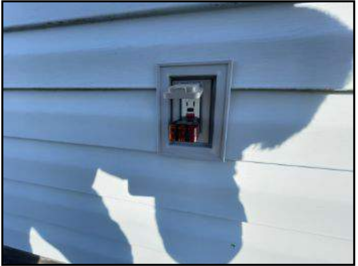
Non-energized outlet at upper exterior balcony
