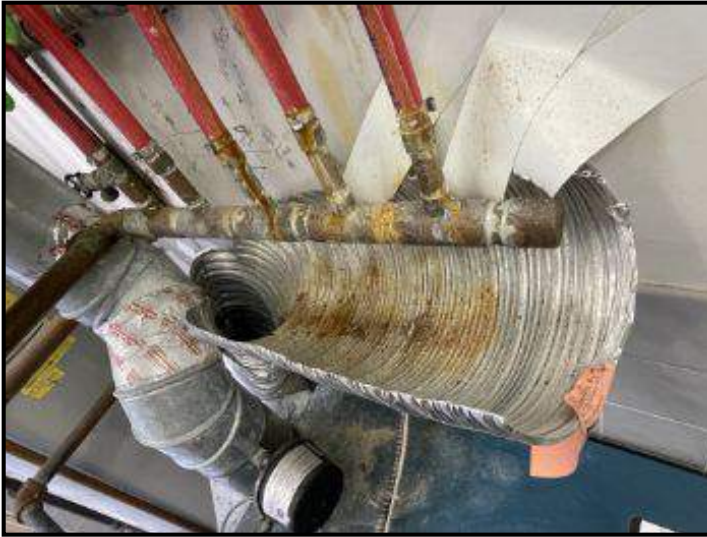
Evidence of possible leak/condensation at manifold above boiler
