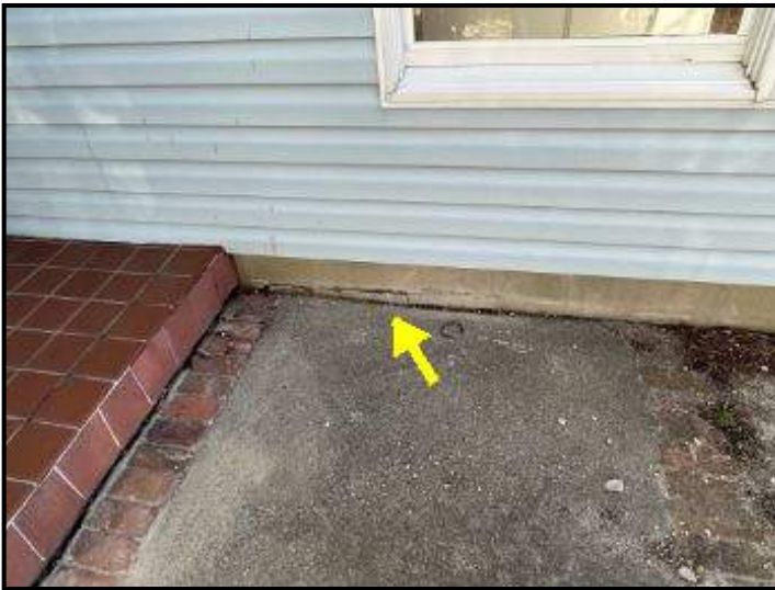
Cracked concrete parging at several areas around the home
