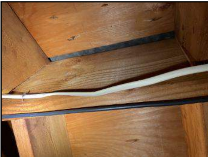
Ridge vent at roof ridge
