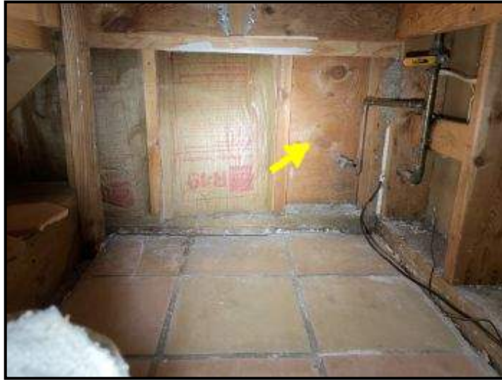
Missing areas of insulation at front exterior wall in closet beneath main staircase
