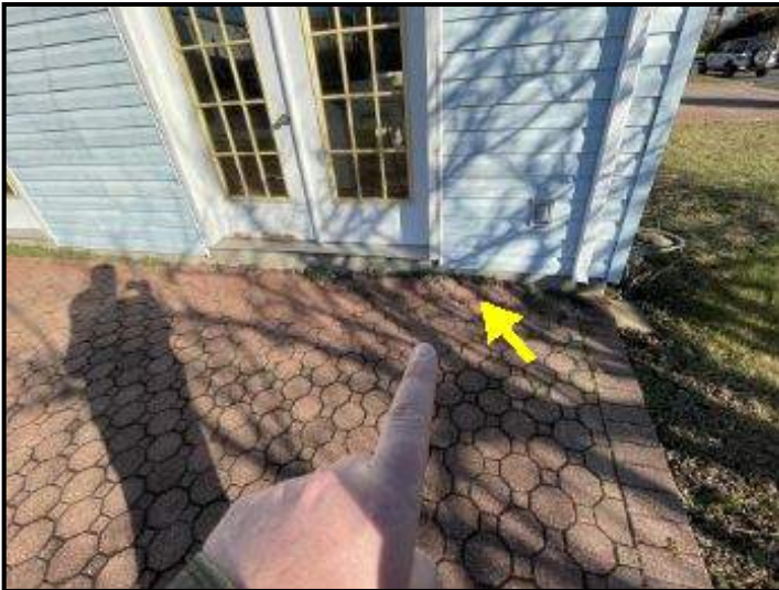
Pavers up-lifted at side paver patio
