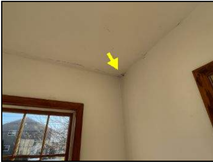
Apparent moisture damage at corner of main living room/office
