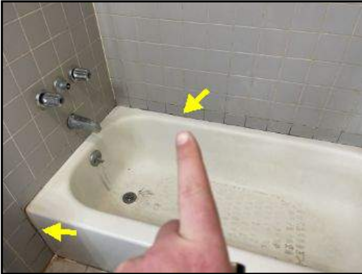
Incomplete caulking around edge and base of tub at upper main bathroom
