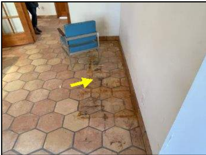
Some staining was observed at areas of tiled flooring at lower level
