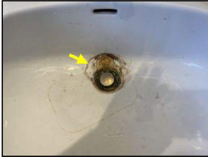
Chipped area of lower main bathroom sink
