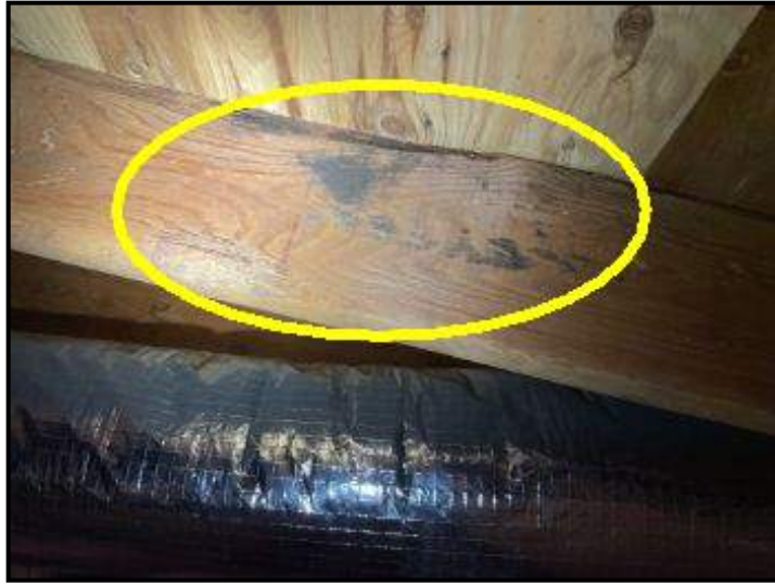
Minor areas of possible mold at roof rafters in attic
