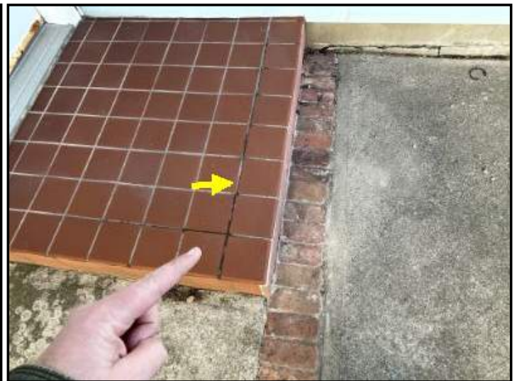
Crack in mortar joint at rear tiled stoop
