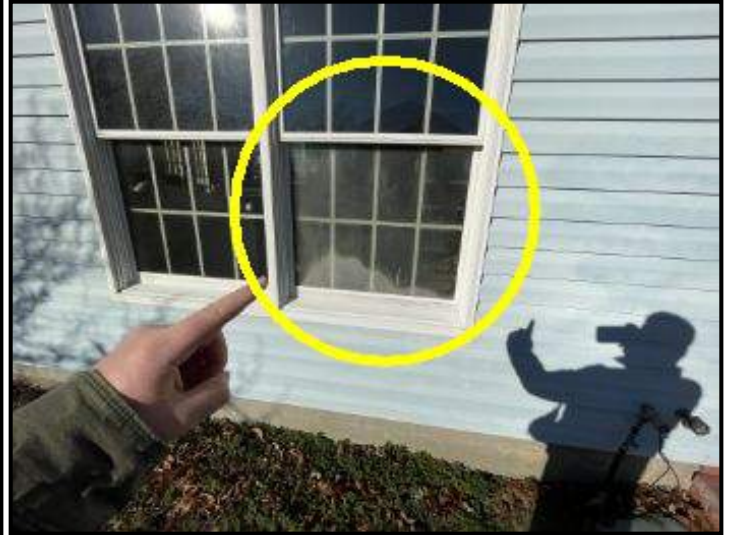
Moisture between panes at front lower window
