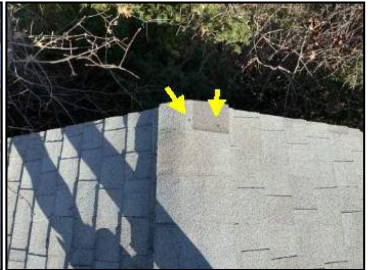
Un-tarred nail heads at edge of roof ridge
