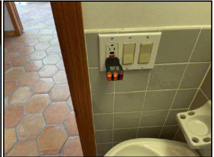
Grounded GFCI outlet at lower bathroom
