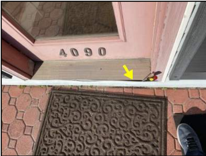
Void at base of front door
