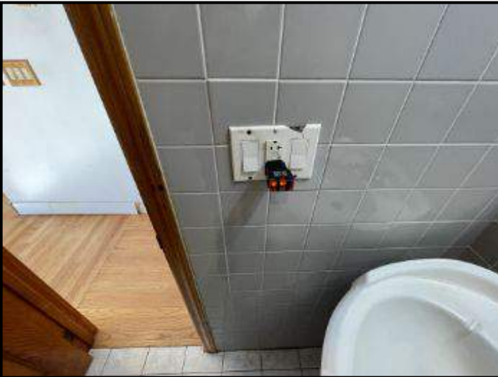
Grounded GFCI outlet at upper main bathroom
