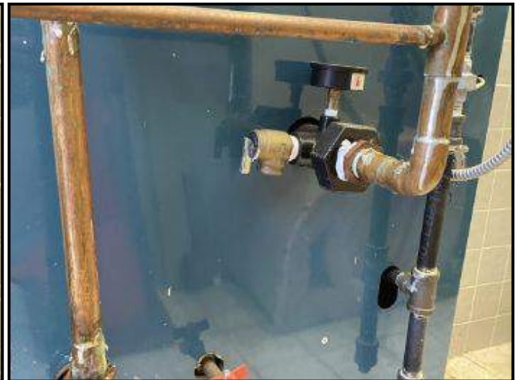
Pressure relief valve not properly installed; no down-line present
