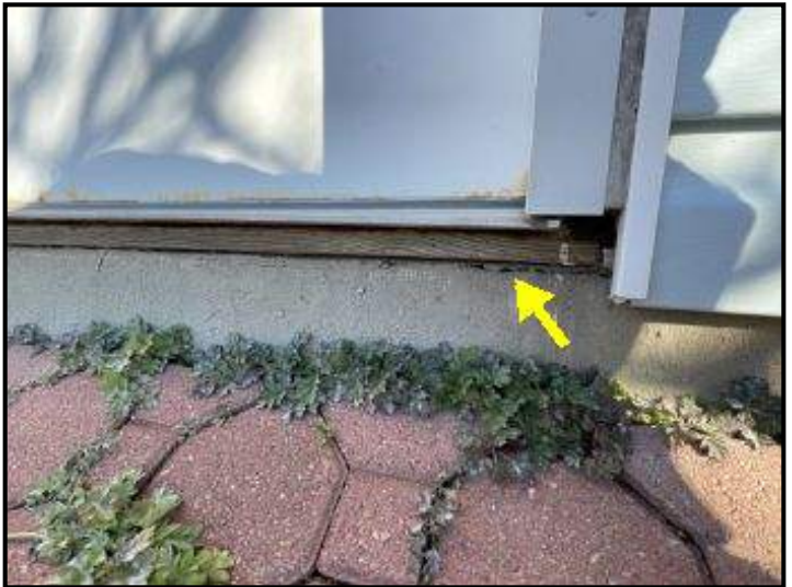
Bare wooden sill at base of side doors
